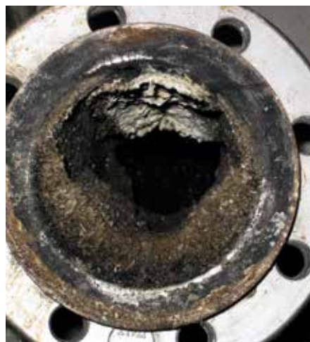
Fig. 4: Struvite deposits in digestate treatment unit
