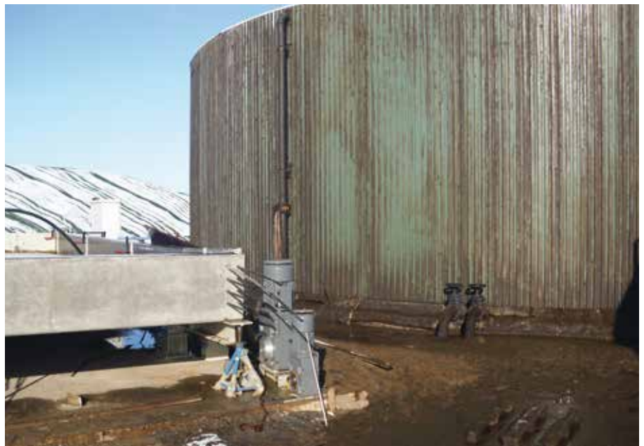
Fig.: Spilt digester content after expansion (“bread dough effect”)
