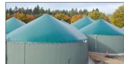
Biogas facility at Hülseberg
